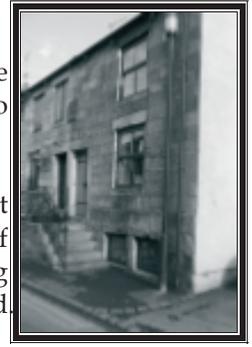
61-62 Church Street had weaving shops in the basement. The ground floor is raised so that windows can be accommodated to let light into the loom shops. There is an identical pattern of windows at the back of the houses. The stone steps would once have faced the other way, leading away from the houses. They have presumably been turned around to allow the road to be widened.
